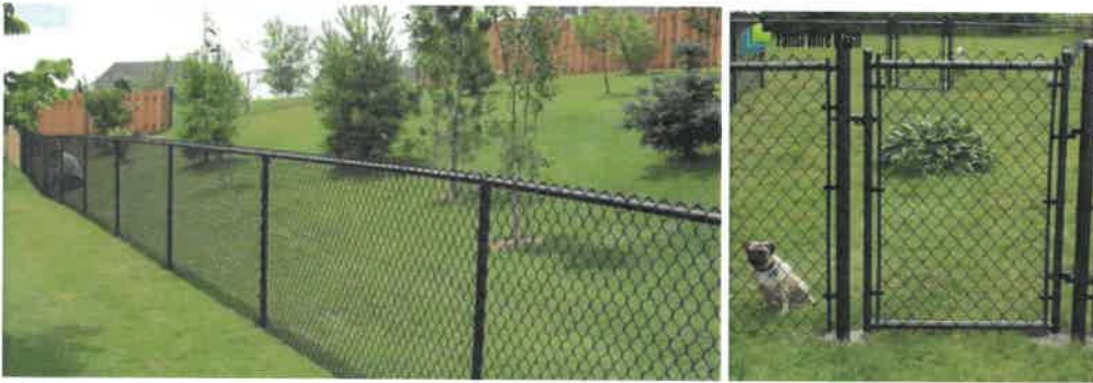
Appropriate coated chain link fence and gate access to open space trails
